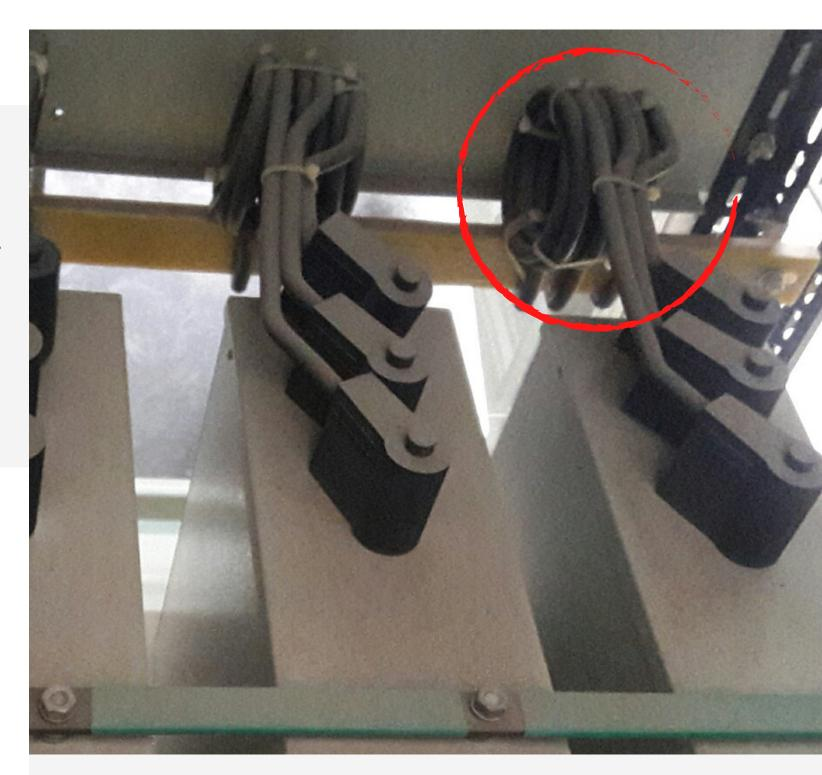
Inrush current coils (Air-core inductors) are used in series with capacitors to limit the capacitors inrush current to a value equal to or less than the capacitor switching rating of the contactor. When a discharged capacitor connects to a voltage source, a huge amount of inrush current flows which is very harmful for capacitors as well as other control equipment connected in panel.
